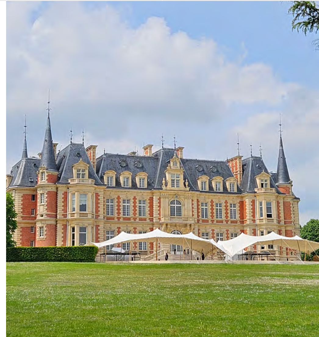
The Serge Kampf Capgemini University at Les Fontaines, France, sits on 52 hectares of parkland and has achieved multiple awards and recognitions for its commitment to sustainability and the protection of biodiversity.
