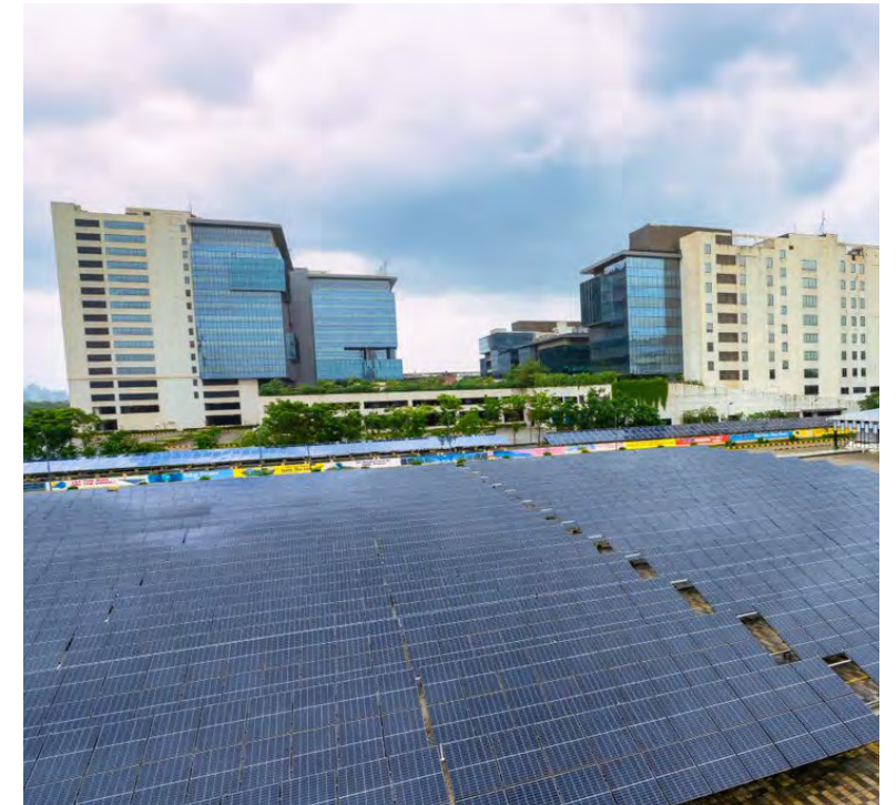
Solar Park, Airoli Campus, Mumbai
